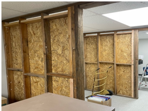
Installation of plywood and the final aspects of building the four walls of the project.
